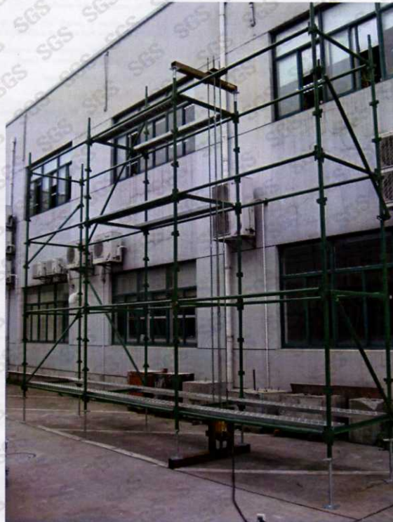
Test arrangement and the erected scaffold
